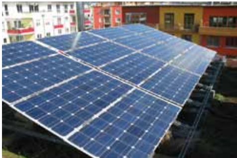
Photovoltaic panels on Green Roof Passivhaus
