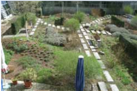
Green roof over Solar Center: Energy plus building; it creates more energy than it uses
